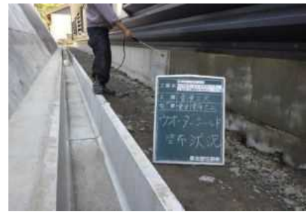
WATER SHIELD塗布状況
